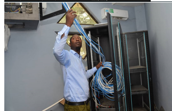
Local Area Network work in progress in the IT server room
