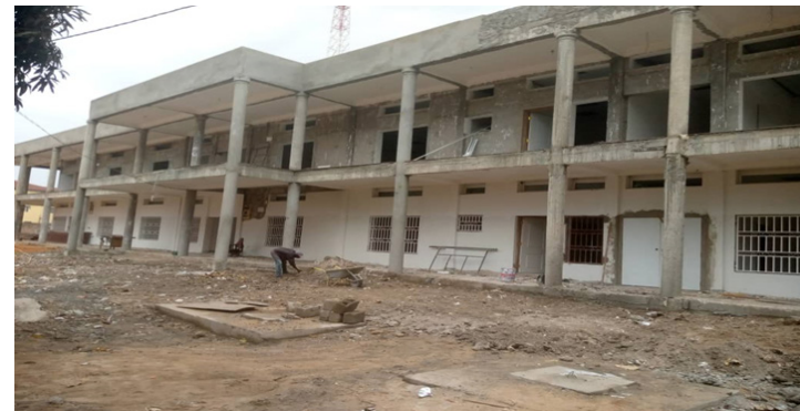
Bundung High Court under construction
